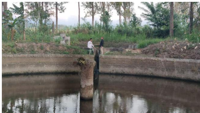
3. Photo of Blombang in the Arrohman Sepawon mosque, which serves as a water reservoir used to irrigate the mosque and the surrounding community.
